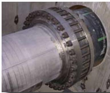
**ESW: Flanged connection between the 36-inch HDPE pipe and stainless steel pipe.**
