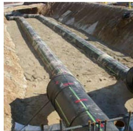
**The 36-inch ESW lines were backfilled using flowable fill poured in lifts.**
