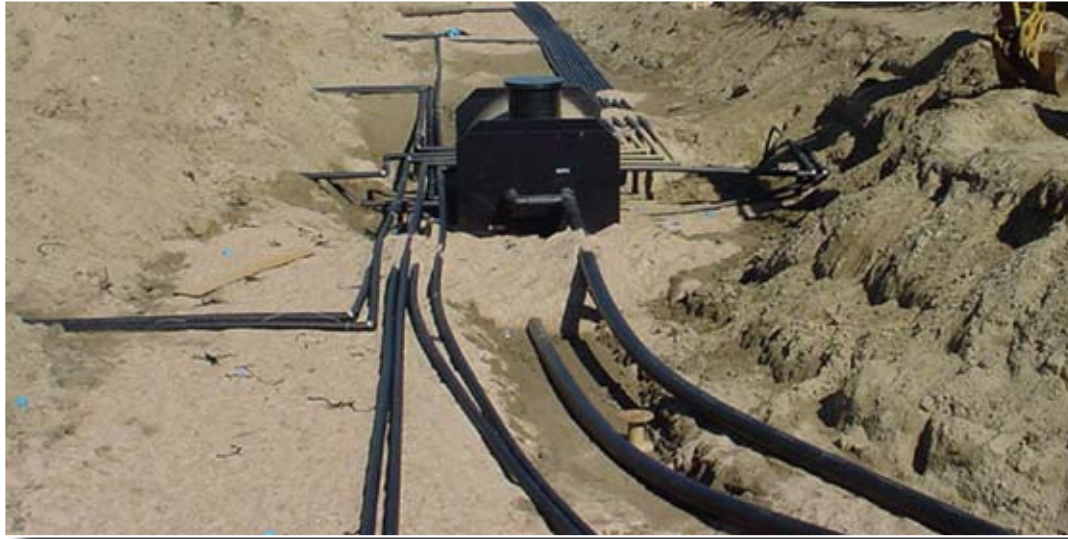
Geothermal well field with ISCO Circuit Maker Vault®
