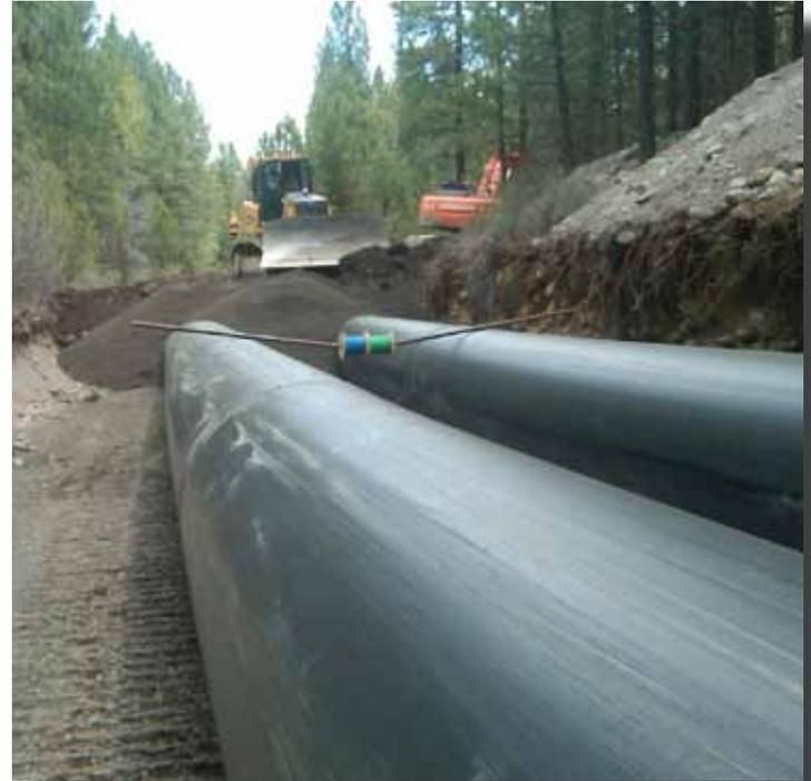
*Two 54-inch HDPE pipelines will be buried to convey water from Whychus Creek to a reservoir.*
