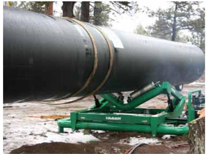
*The pipe is fused together to create a leak-free system.*
