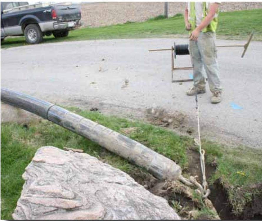
*HDPE pipe installed using horizontal directional drilling.*
