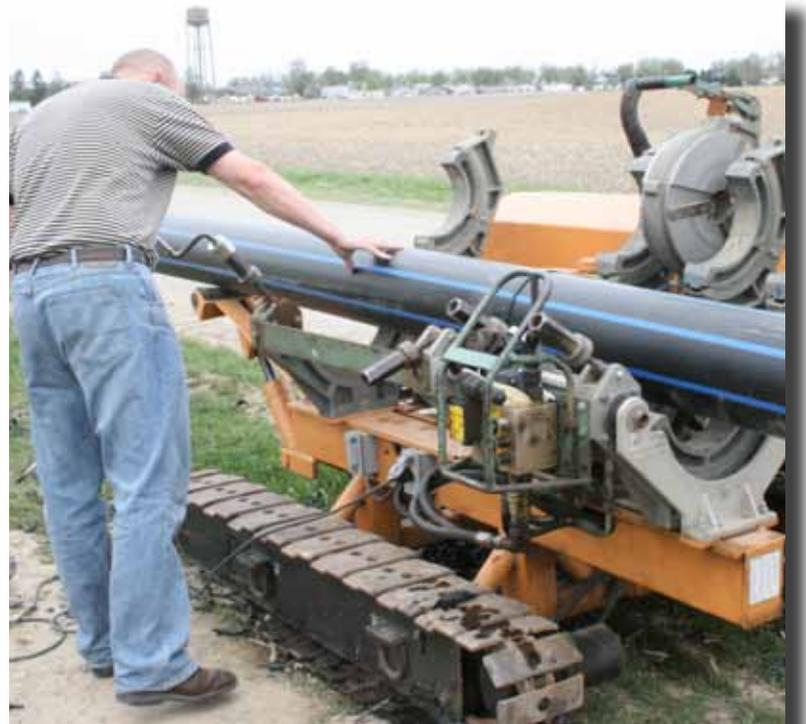
*HDPE pipe placed on the fusion machine.*
