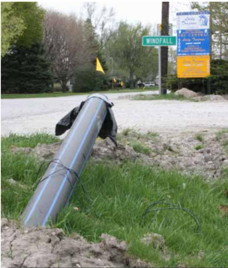
*By installing the pipe using horizontal directional drilling, there is no need for open cut, saving the city money.*
