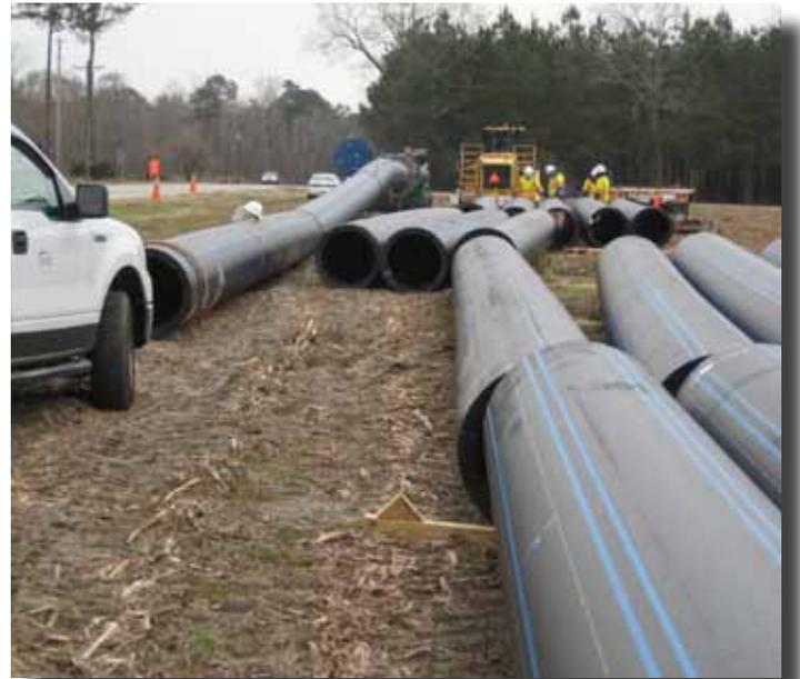
*Pipe onsite being fused to get ready for installation via horizontal directional drilling.*
