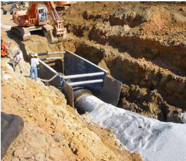
Wilson and Coronaca Creek Trunk Sewer Replacement Installation
