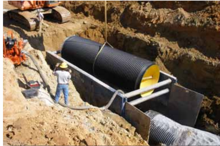
Phase I Installation of HDPE Pipe in Greenwood, SC
