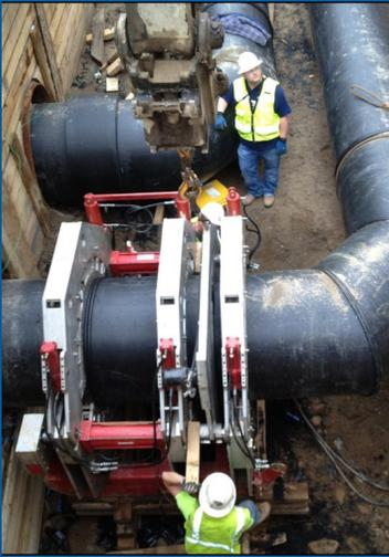
“Specialized in-hole fusion equipment, special fitting fabrication ability, and knowledge of the product and specification.”
