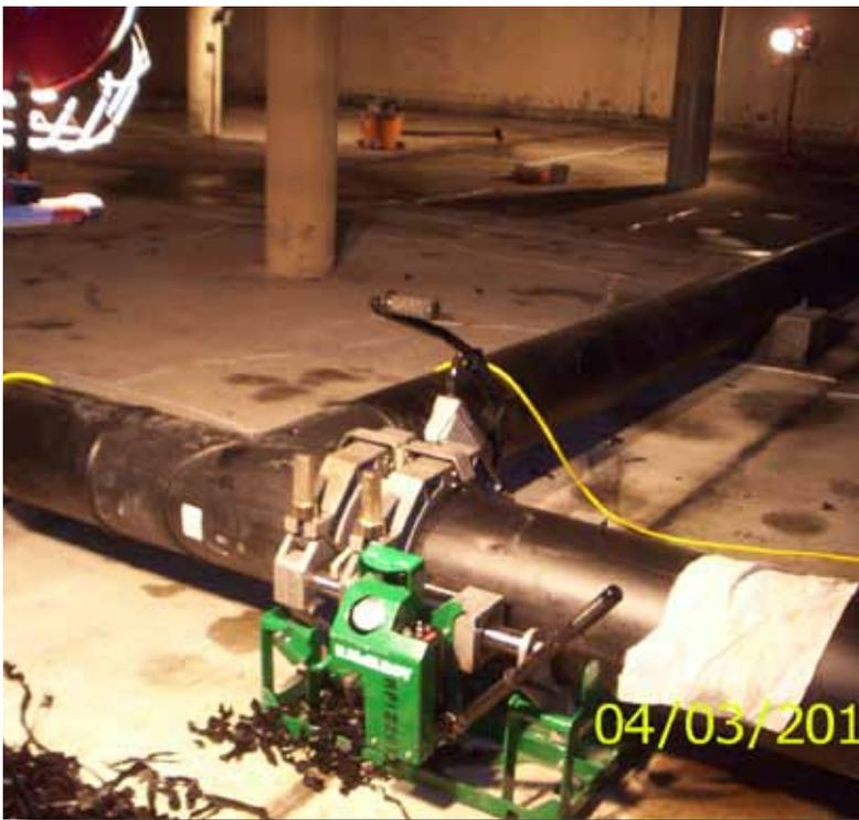
*HDPE pipe being fused and installed inside the storage vault.*
