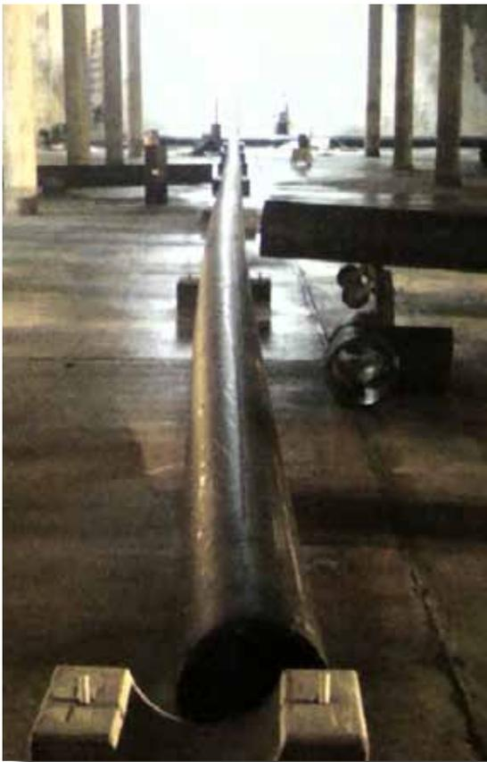
*HDPE pipe inside the storage tank waiting to be fused.*
