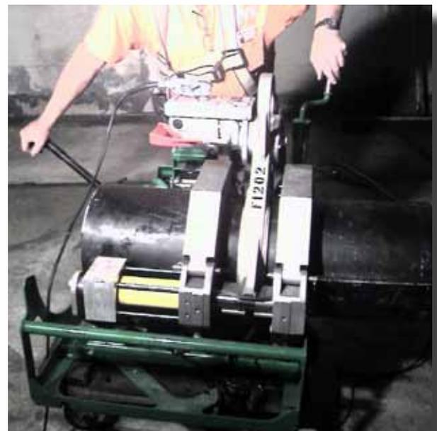
*Pipe being fused with McElroy fusion unit inside the water tank*
