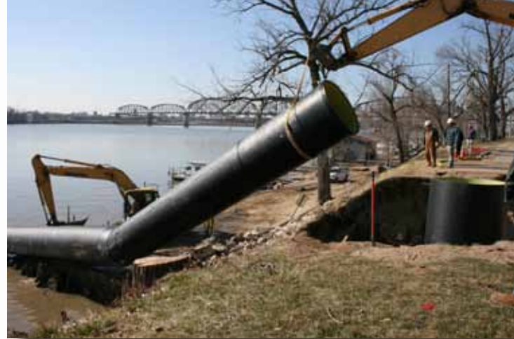
Large -diameter pipe lowered into trench to connect to manhole
