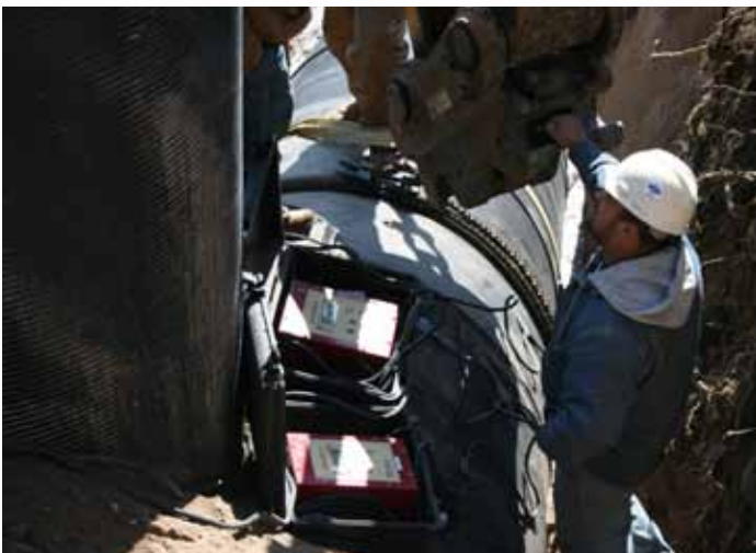
Large-diameter profile pipe joined to manhole using electrofusion
