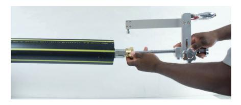
1. Insert the scraper into the pipe/fitting.
