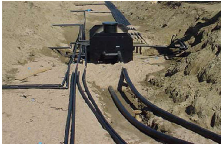
Geothermal well field with ISCO Circuit Maker Vault®
