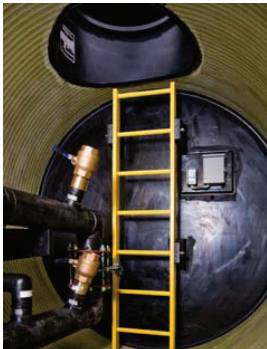
Geothermal well field with ISCO Circuit Maker Vault®
