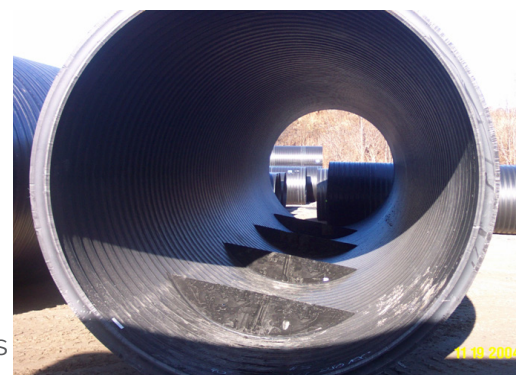
Baffles are placed off center from the invert or flowline of the culvert and remain on one side of the culvert and do not alternate.
