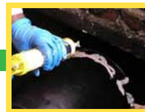
4 Silicone can be applied lightly to the male ends. The second piece is lowered into position and threaded together to the first piece using a strap-wrench. The joint automatically self seals.
