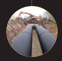
3. With a Mannings "n" value of 0.009, Spirolite® maintains long-term flow with less friction — reducing pipe sizing and slope requirements.
