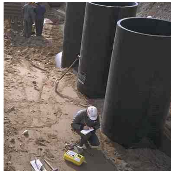
FIGURE 3B: MEASURING EMBEDMENT DENSITY
