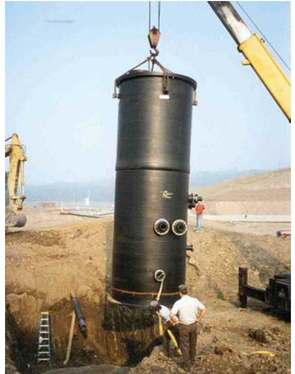
FIGURE 1A: PLACING MANHOLES
